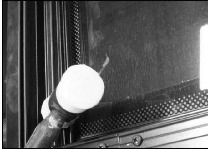
Figure 3-23. INSTALL HIDDEN FRAME CLIPS
