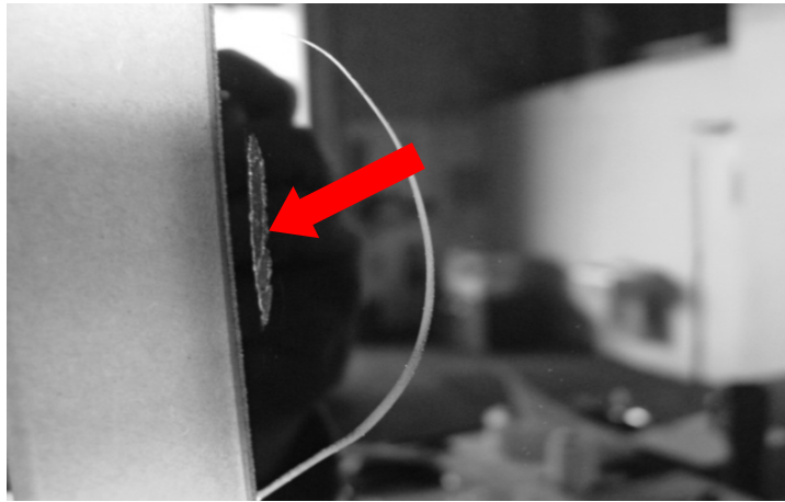
FIGURE 2-2: DEFECTS IN THE GLAZING
