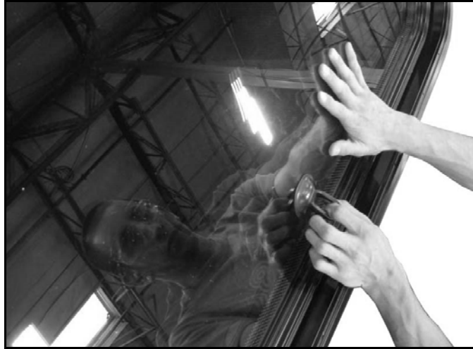
Figure 3-12. Pull Window Liner Using Suction Cup
