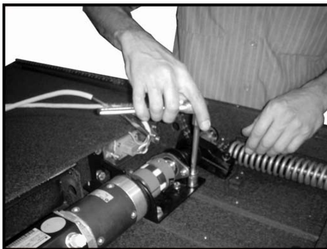
FIGURE 2-4: INSTALLED MOTOR DRIVE ASSEMBLY
