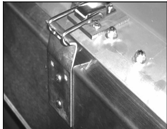
FIGURE [5]: LATCH AND STRIKER
