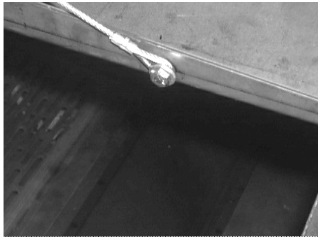
FIGURE [3]: CABLES ON BOTH SIDES OF ROLLSTOP
