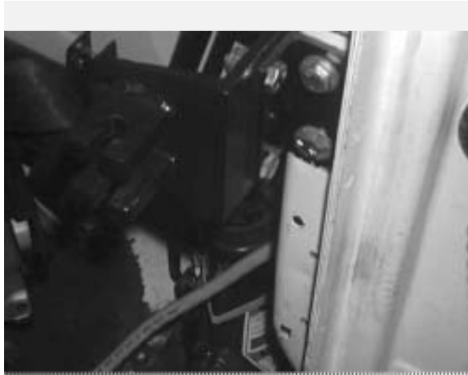
FIGURE [3]: CLEVIS & ALUMINUM BRACKET INSTALLED
