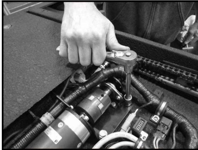
FIGURE 2-5: INSTALLED MOTOR DRIVE ASSEMBLY
